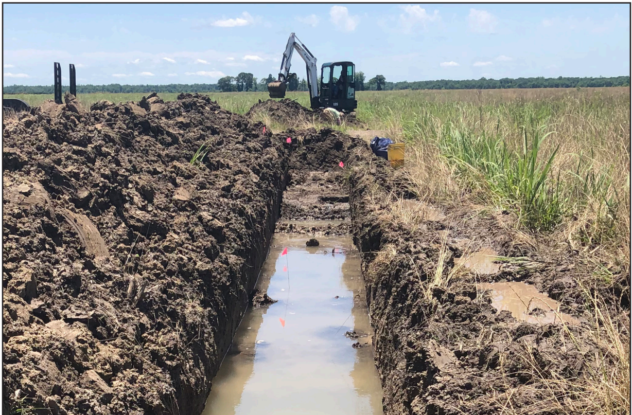
Figure 6.1. Photo of mechanical excavations within the Buena Vista Cemetery, facing southwest.
