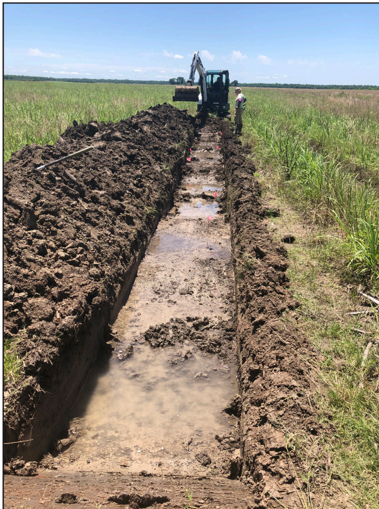
Figure 5.1. Photograph of the trenching process on the Buena Vista Cemetery, facing southwest.
